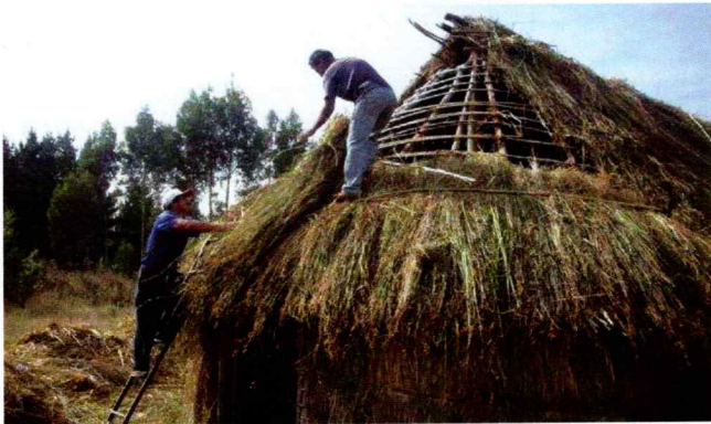
Repairing the roof.
