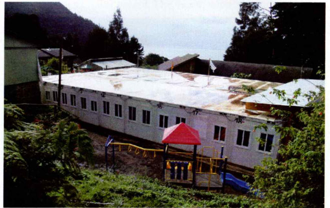
One of the two modular blocks.
