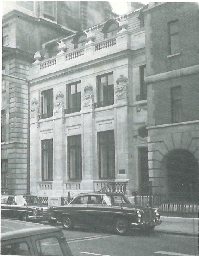
The new Chilean Embassy and Consulate building in London, at 12 Devonshire Street, W.1.
