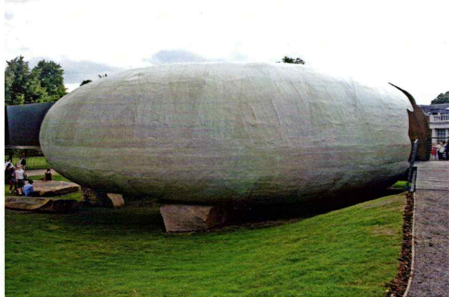
View from the Ring Road of Hyde Park of the Pavilion supported on the limestone blocks.
